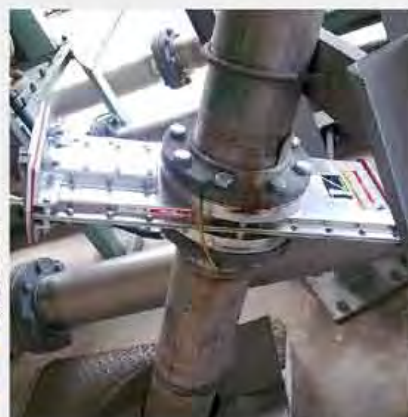
Hand crank Quantum Orifice Gate with ANSI flange
