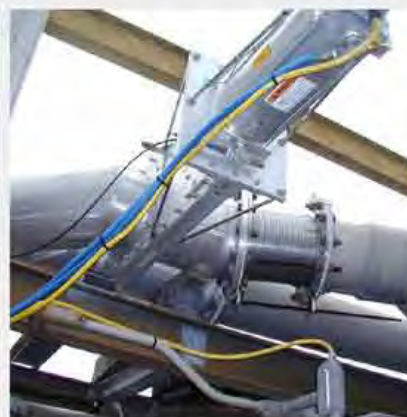
12" (305mm) Quantum Orifice Gate handling polyethylene resin powder
